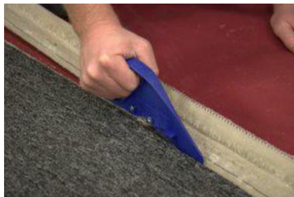
Figure 3-3: Trimming Carpet
