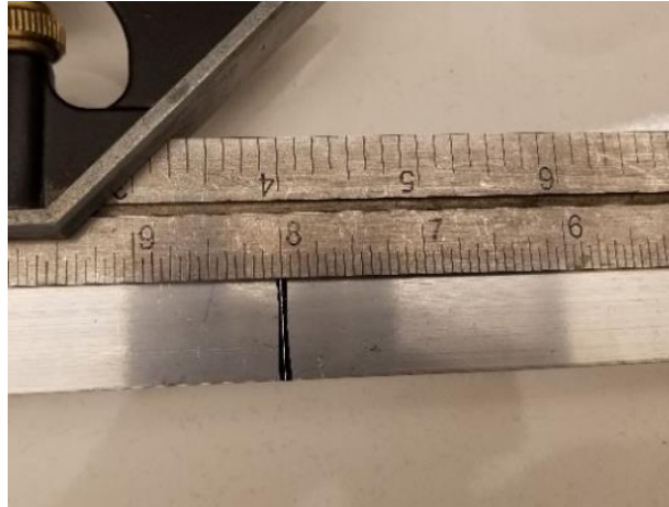
Figure 5: Marking 8 in. on Vertical Tube
